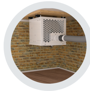
• in the basement
